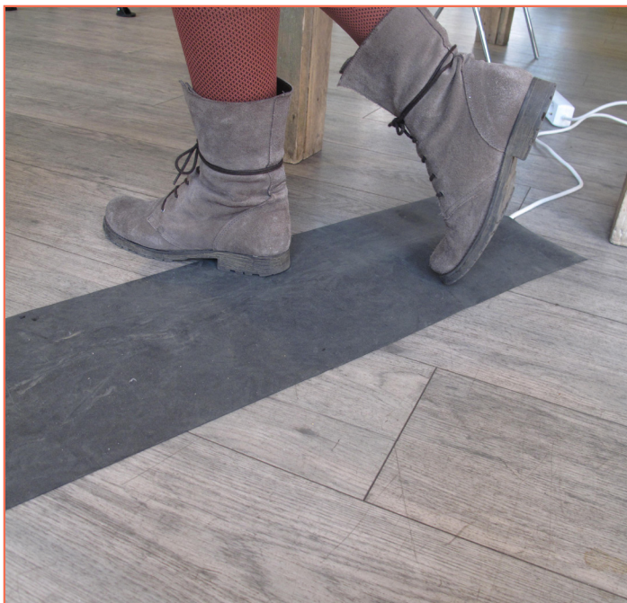
Safe: extension cords covered with rubber mats
